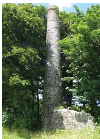
Chimney, Holmbush Mine
