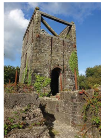
Bailey's Shaft engine house, Hingston Down Mine
