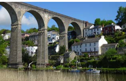
Calstock Viaduct towers over the river
